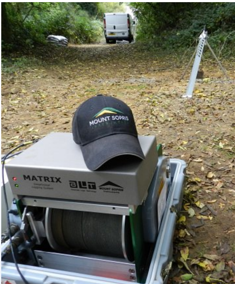
Matrix Logger installed onto MX Winch.
